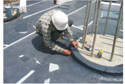
Construction site HSBC Bank Egypt
